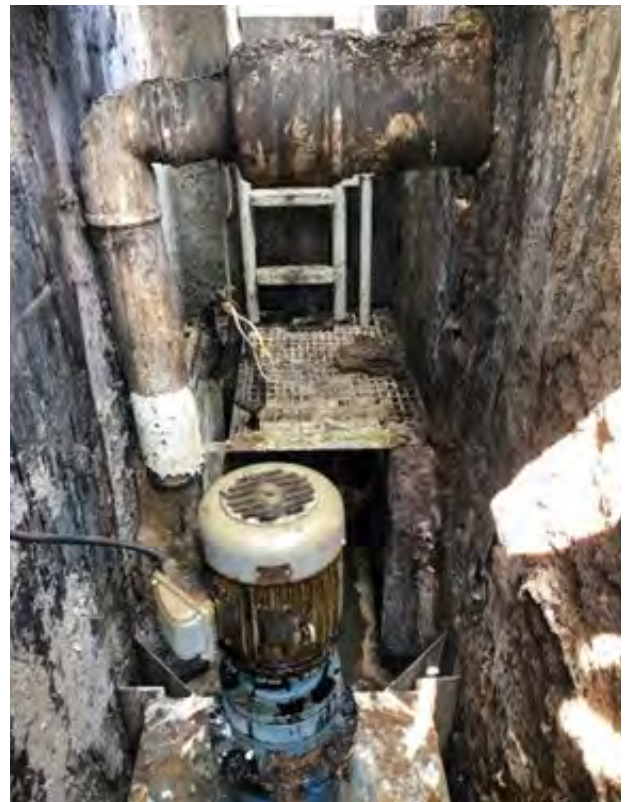
LINE 59 STATE ROAD PUMP STATION $400,000
