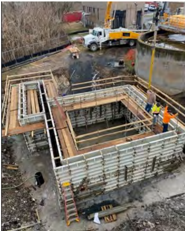
LINE 57 WASTEWATER 3B PROJECT $2,000,000
