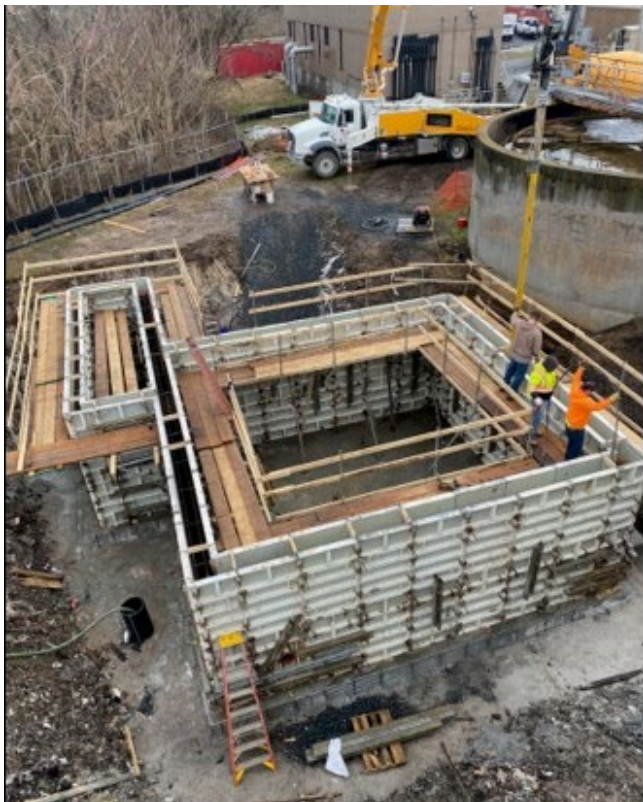
LINE 57 WASTEWATER 3B PROJECT $2,000,000
